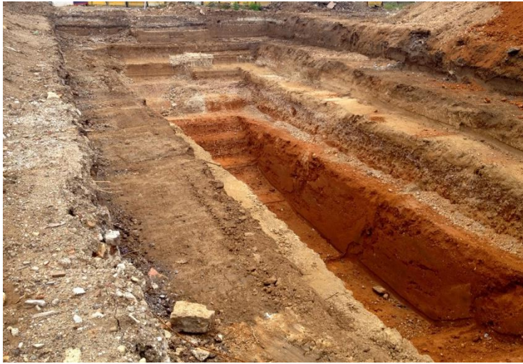
FIGURE No. 2: EXCAVATING THE SOIL FOR EXAMINATION (SOIL ANALYSIS PIT)
