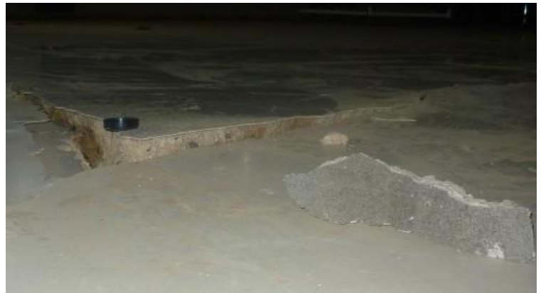
FIGURE No. 20: PAVING RAISED BY WATER UNDERGROUND
