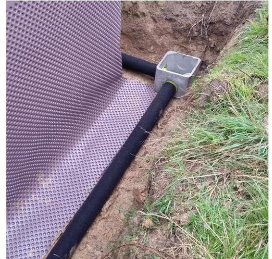
**FIGURE No. 18: CHANGING DIRECTION USING AN INSPECTION BOX**
