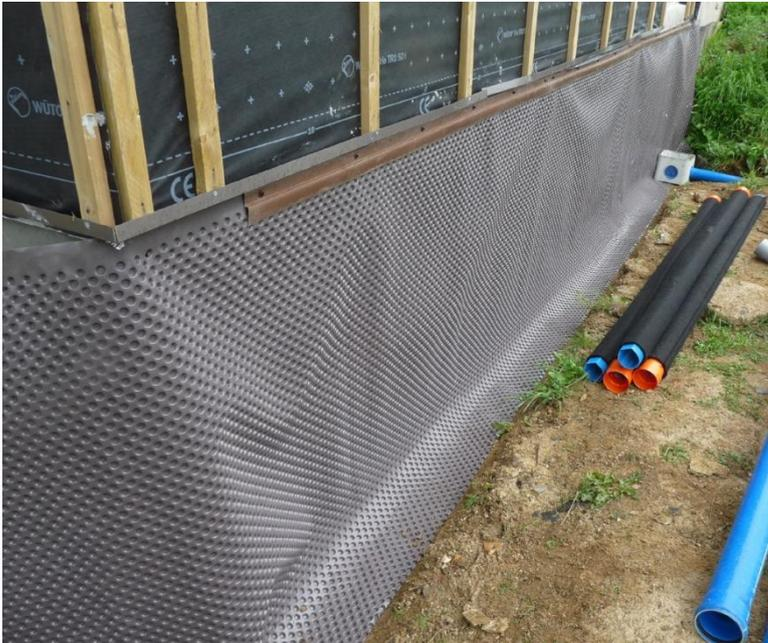
**FIGURE No. 12: USING AN EMBOSSED FILM TO PROTECT THE SEAL**
