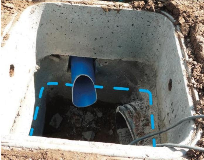
**FIGURE No. 1: CONNECTING THE DRAIN NETWORK TO AN OUTLET**
