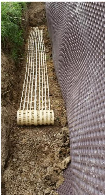
**FIGURE No. 27: USING A WARNING MESH**
