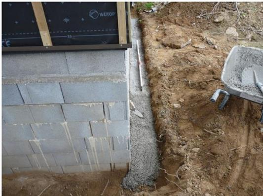
**FIGURE No. 8: CREATING THE THIN CONCRETE CHANNEL & CHECKING THE SLOPES**
