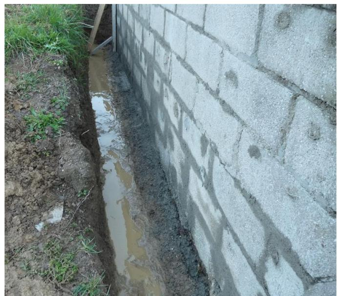
**FIGURE No. 5: RE-POINTING THE FOUNDATION FACING**
