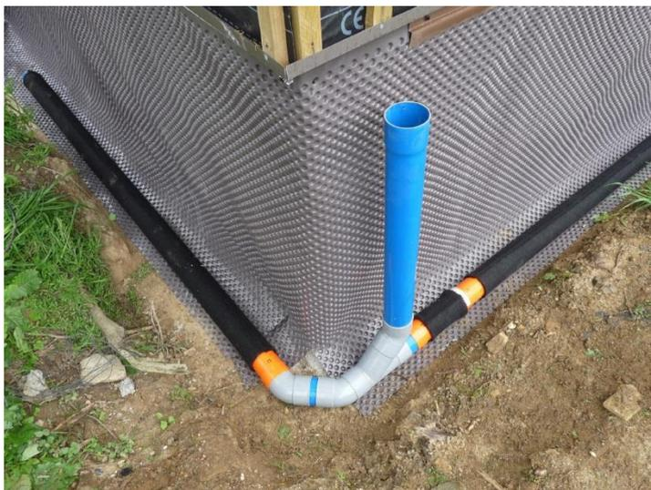
**FIGURE No. 19: CHANGING DIRECTION USING TWO 45° BENDS PVC Ø100**
