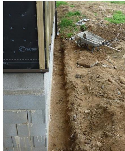
**FIGURE No. 7: CLEANING AND WIDENING THE TRENCH**
