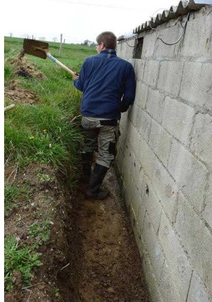
**FIGURE No. 3: REMOVING THE FOUNDATIONS USING AN EXCAVATOR AND FINISHING OFF USING A HAND SHOVEL**
