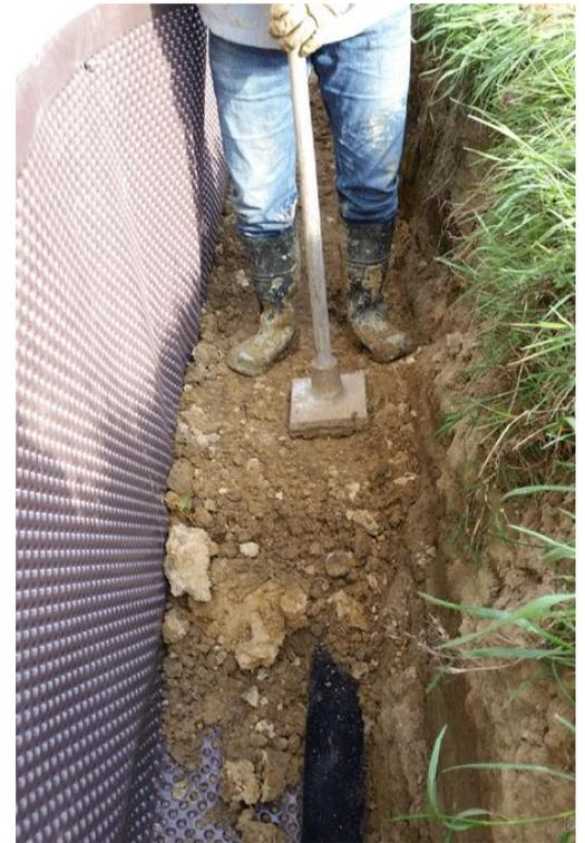
**FIGURE No. 26: MANUAL DAMAGE TO THE LAYERS OF BACKFILL**
