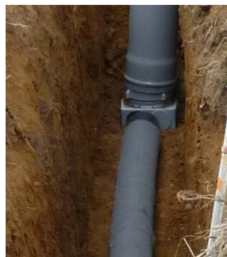
FIGURE 18: LOOP AND DISTRIBUTION MANHOLE
