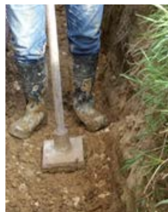
FIGURE 24: MANUAL COMPACTION OF THE BACKFILL LAYERS
