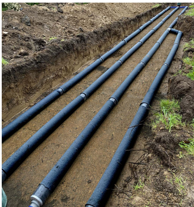
FIGURE 11: EXAMPLE OF INFILTRATUBE INSTALLATION
