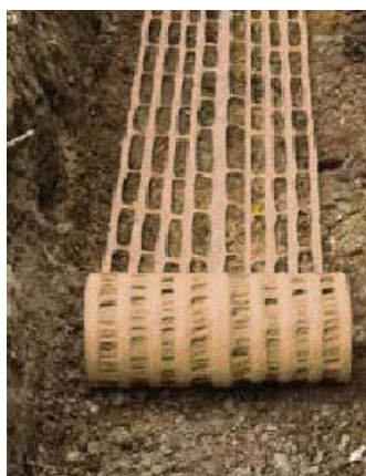
FIGURE 23: INSTALLATION OF THE BROWN WARNING MESH
